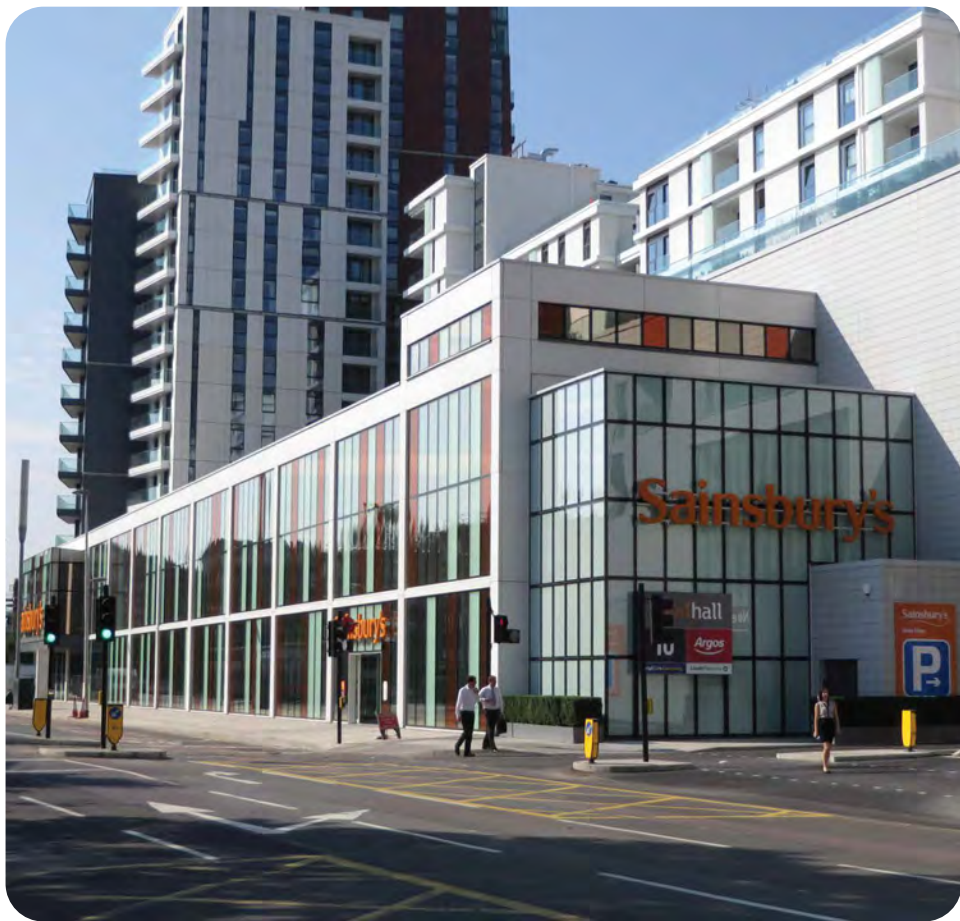
Sainsbury's and Barratt London partnership, Nine Elms
